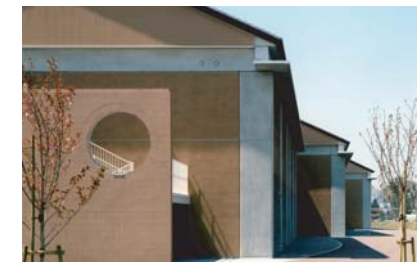
Detail : Edge of eaves (Practical Training Building)
